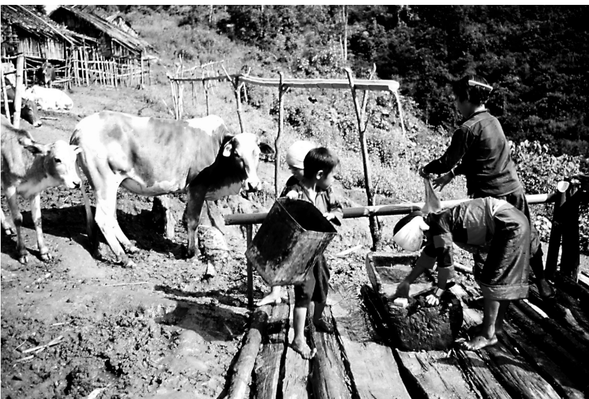
Fig. 2: Bamboo aqueducts raised on forked wooden posts, bringing water into the village; it is raised sufficiently high above the ground to permit cattle to move freely underneath it. The girl at right washes clothes in a large carved-out wooden trough.
