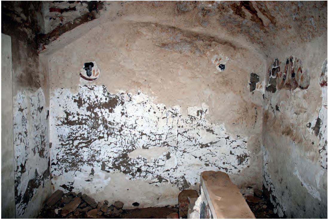
Abb. 13: Erdgeschoss, 2. Raum, Westwand; 2008
