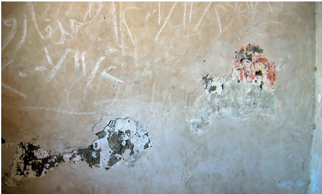
Abb. 10: Erdgeschoss, 1. Raum, Detail Westwand; 2005
