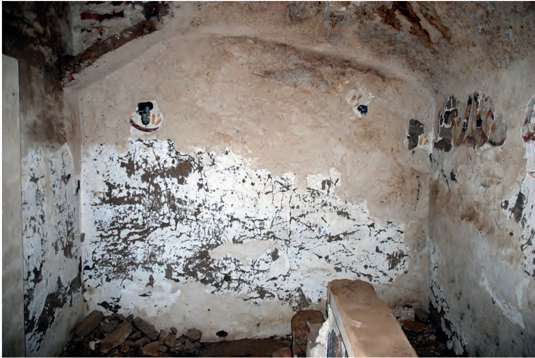
Abb. 13: Erdgeschoss, 2. Raum, Westwand; 2008
