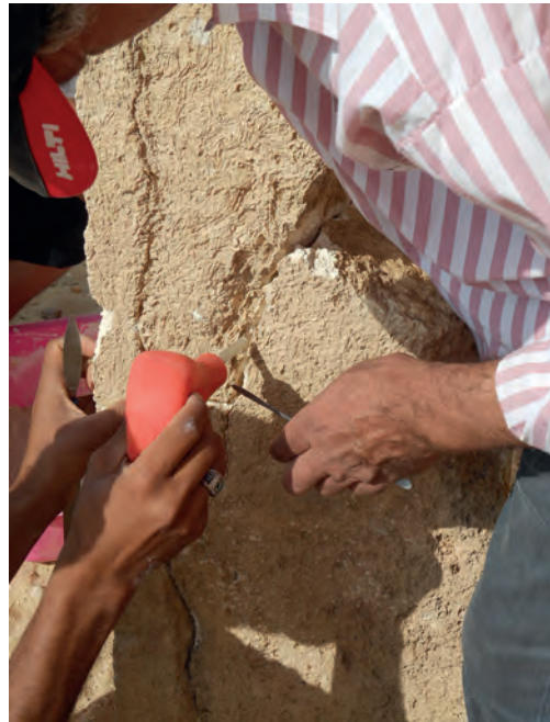
Fig. 13: Closing gaps with the help of lime mortar; 2015
