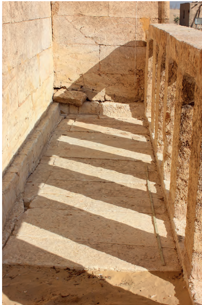
Fig. 5: Preserved pavement between naos and balustrade; 2015
