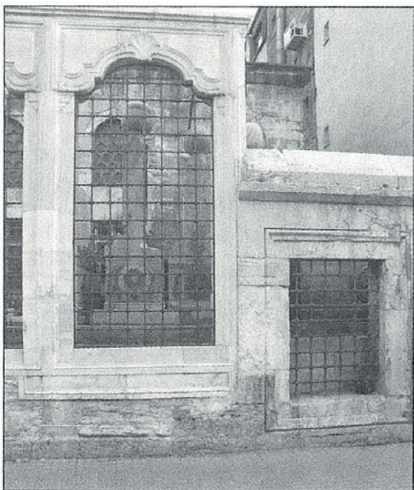
Fig. 74: Detail of the Koca Sinan hazire openings.
