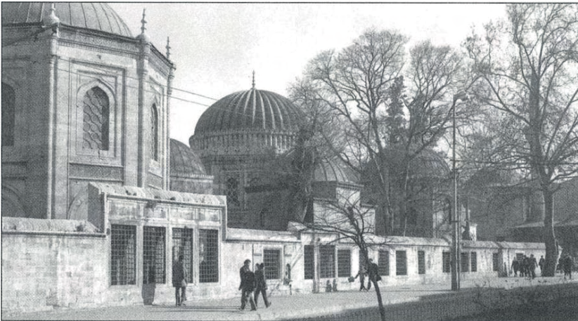
The Şehzade precinct wall on the Divan axis. Fig. 68: South-eastern wall and mausoleums.
