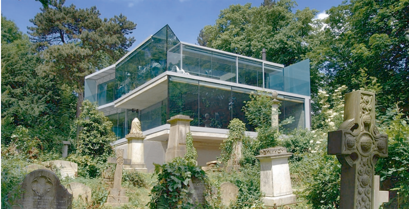
Fig. 5: Eldridge London Architects + Designers, House in Highgate Cemetery, Swains Lane (Image: Lyndon Douglas 2008, © Eldridge London).
