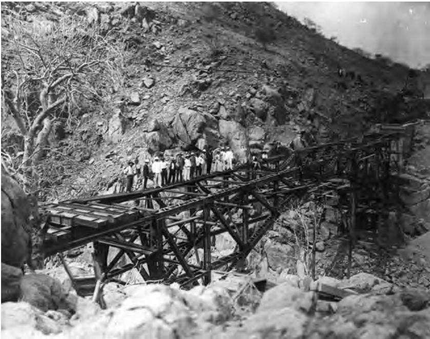
Ill. 6 Railway construction in southern Angola, photo: Carl Singelmann, 1911
