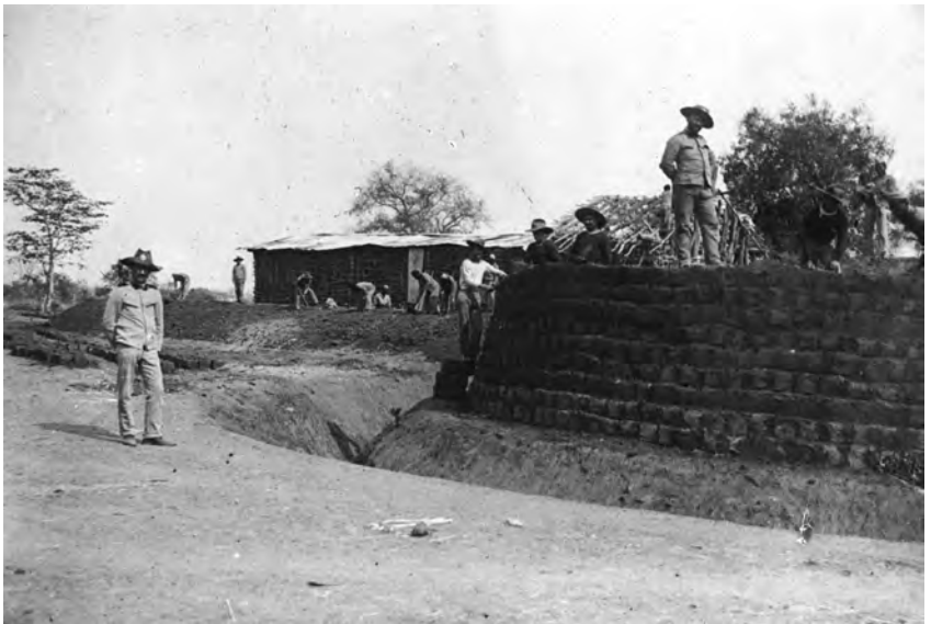
Ill. 3 Construction of a Portuguese fort, photo: Carl Singelmann, 1911
