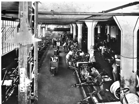
Abbildung 13: Chassis-Montagelinie in Highland Park (1914)
