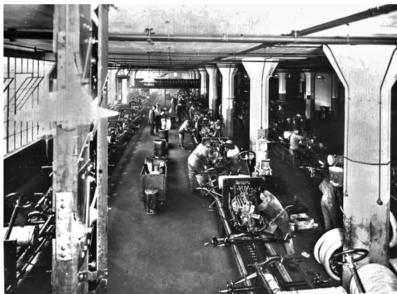
Abbildung 13: Chassis-Montagelinie in Highland Park (1914)
