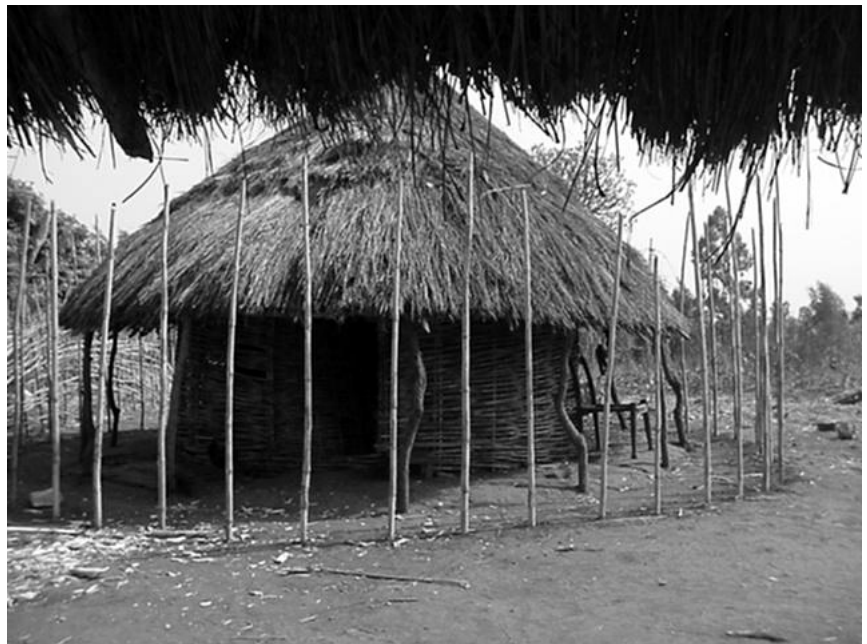
Fig. 7: Building an external ring to enlarge a kitchen and transforming it in a main house. Gundul (Asosa).
